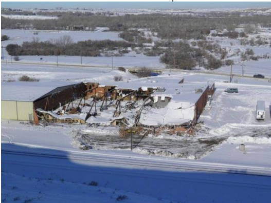
The destroyed Central Building, home of Prairie Gleaners
