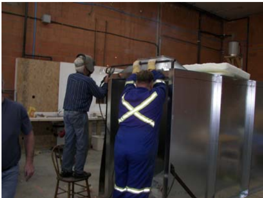
Welding some of the Frame
